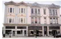
Post-1880s commercial buildings
